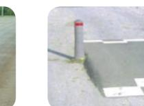
Bollards installed in conjunction with environmental obstacles to ensure that the cars cross the obstacle with both wheels whilst two-wheeled vehicles can pass without crossing the obstacle.
